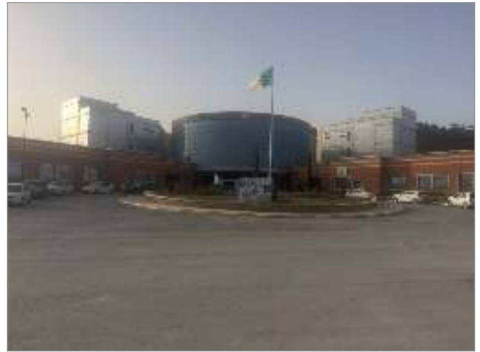
Figure 2: Oncological Surgery Center/ Batna-Algeria
